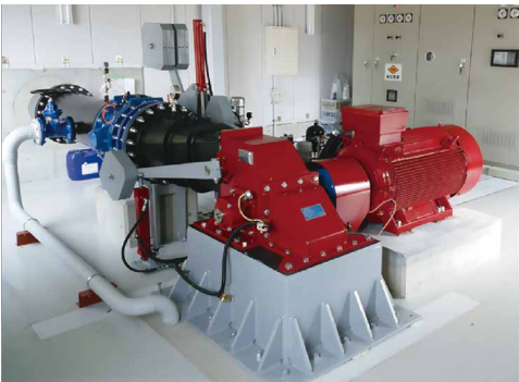
Water turbine generator (rated capacity: 136 kW)
