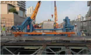
Deck slab removal with shared use of dedicated machinery
