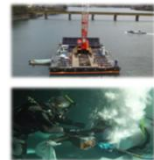
Diving Works Underwater Structure Repair & Renewal
