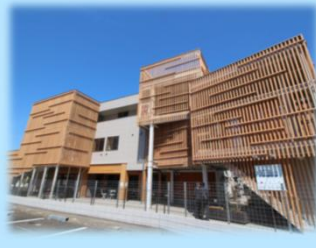
Construction of a Wood-Frame Support Facility for People with Disabilities (Tobishima Corporation × Wood Engineering)
