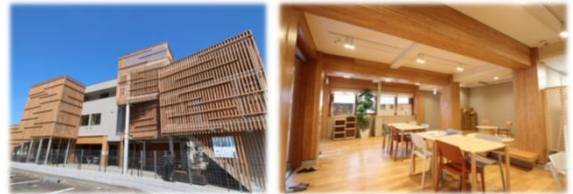
Collaboration Example: Construction/Development of a Wood-Frame Senior Care Facility
