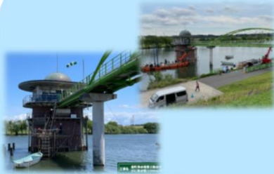
Seismic Retrofitting of a Water Treatment Plant (Tobishima Corporation × Tequanauts)
