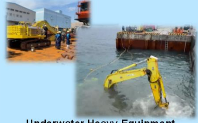
Underwater Heavy-Equipment Construction Work at a Port (Sugita Construction × Kyokuto Construction)
