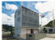
Ogasawara Coast Guard Station-Related Facility Construction
